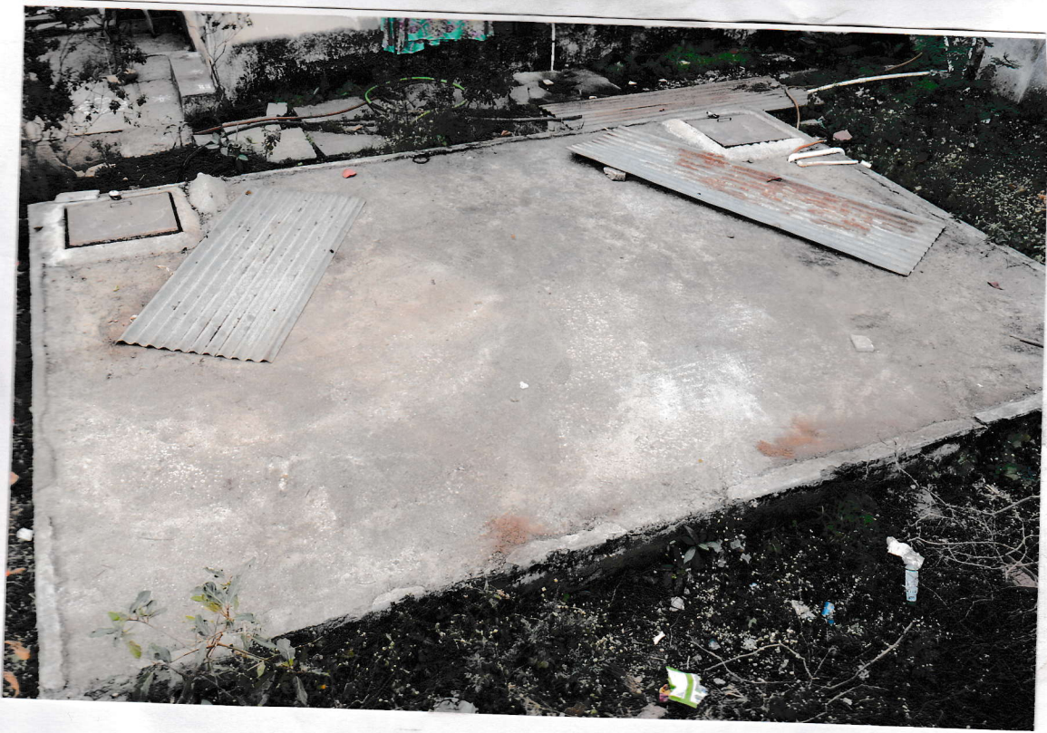
7-1-4 Water Conservation Facilities .
