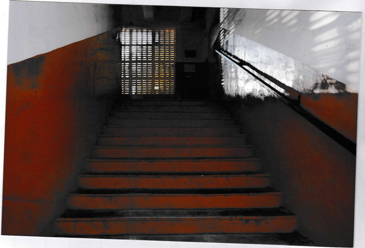
7.1.7 Ramp - Rails for Disabled students.
