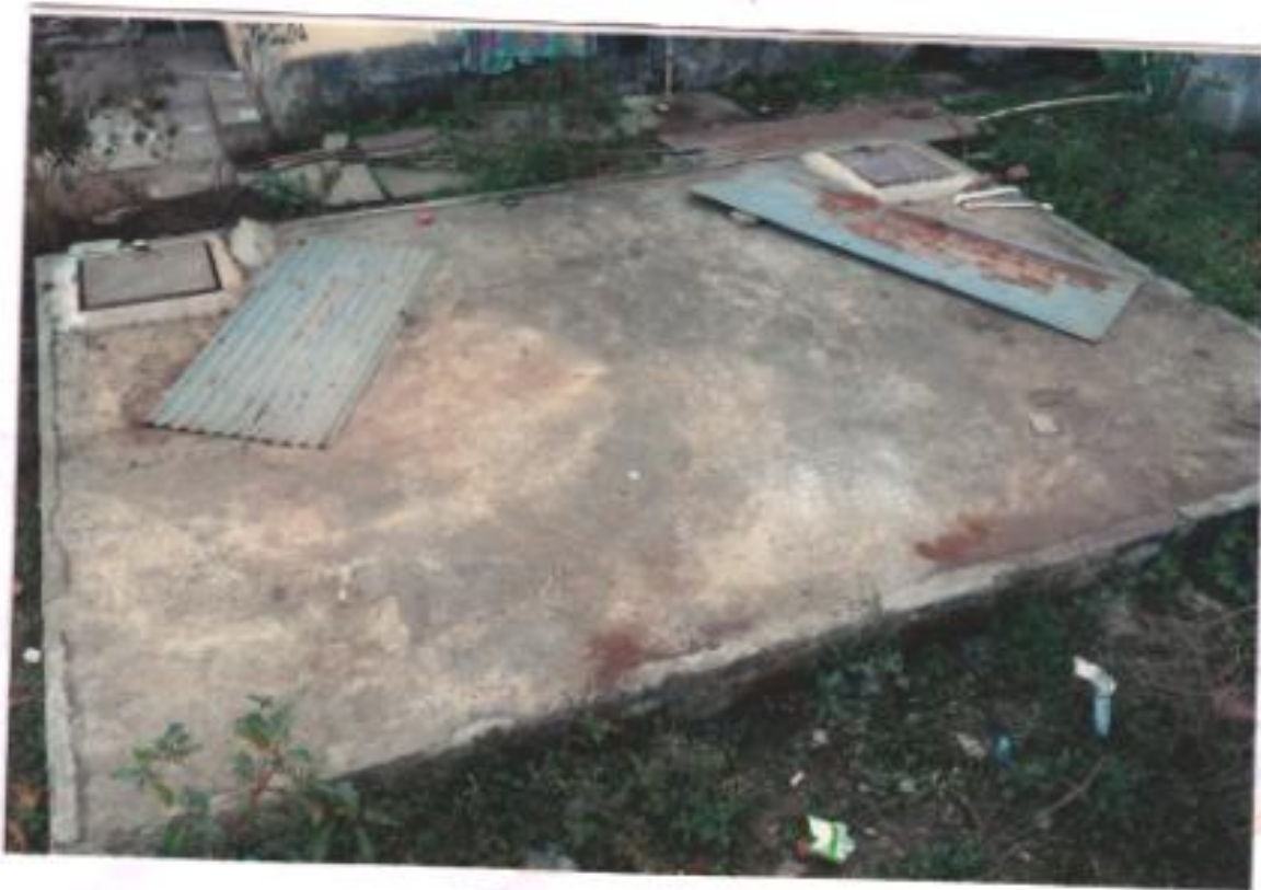
7.1.4 Water conservation Facilities .
