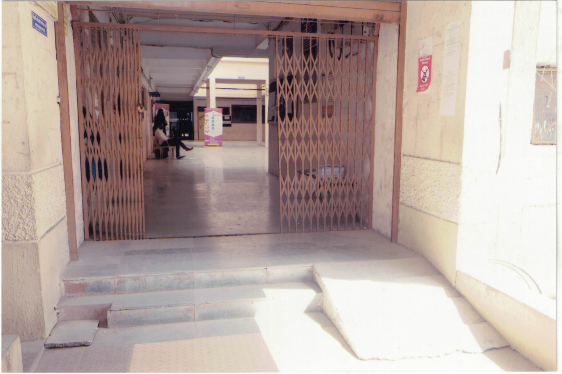
7.1.5 Ramp to enter in the college
